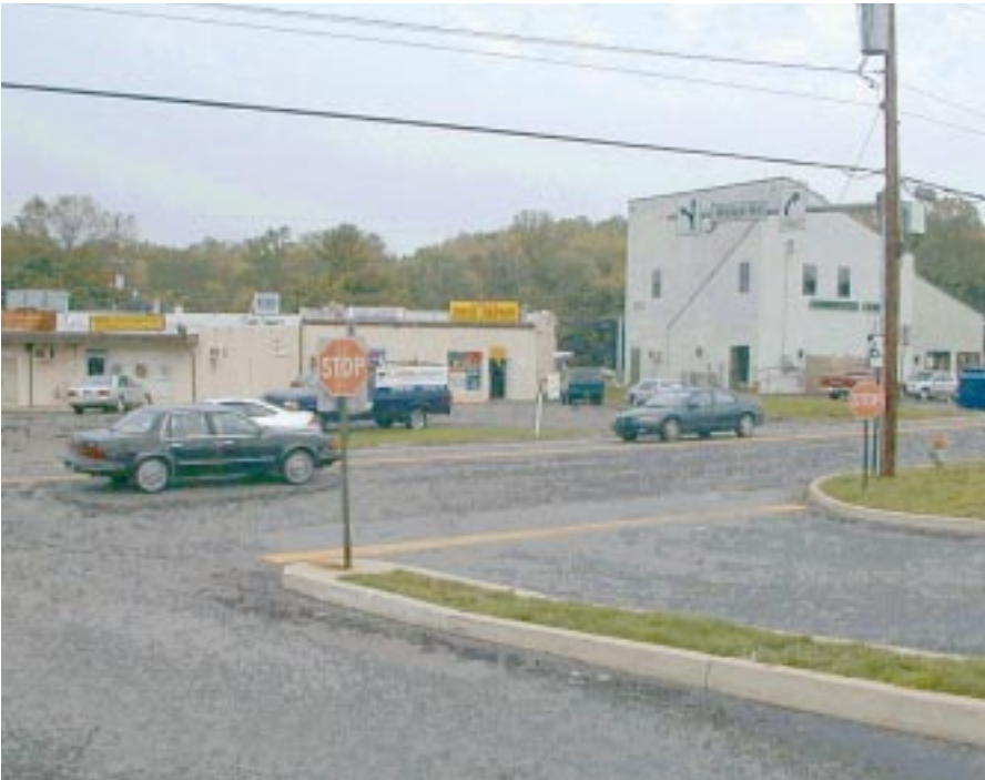
When access drives are located too close to intersections, confusion about who has the right-of-way has the potential to cause accidents.
