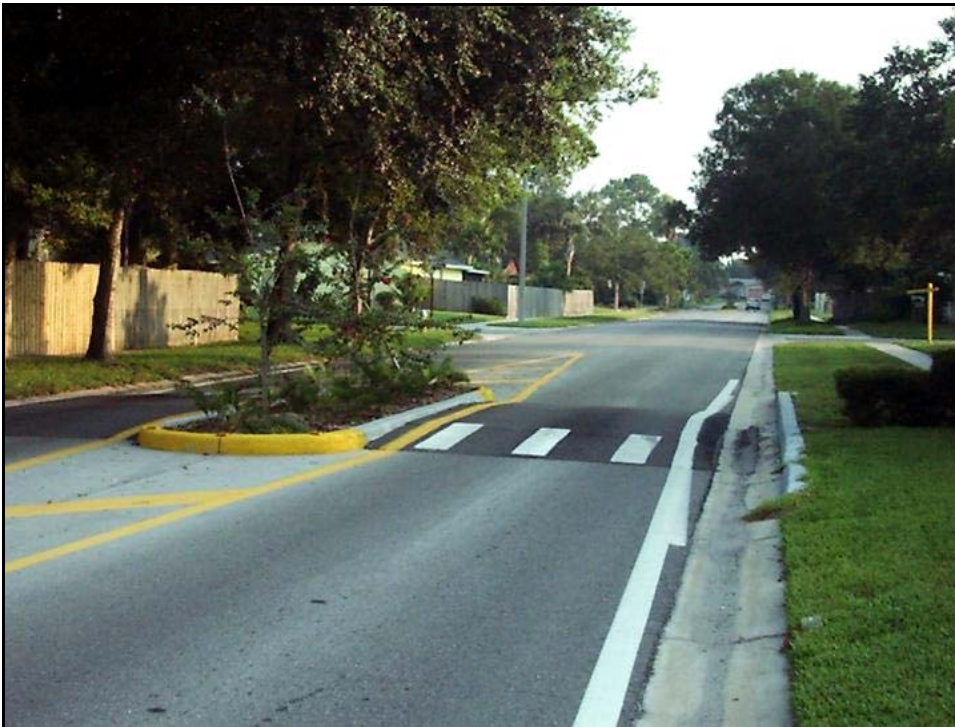
Island combined with speed hump to further reduce speed
