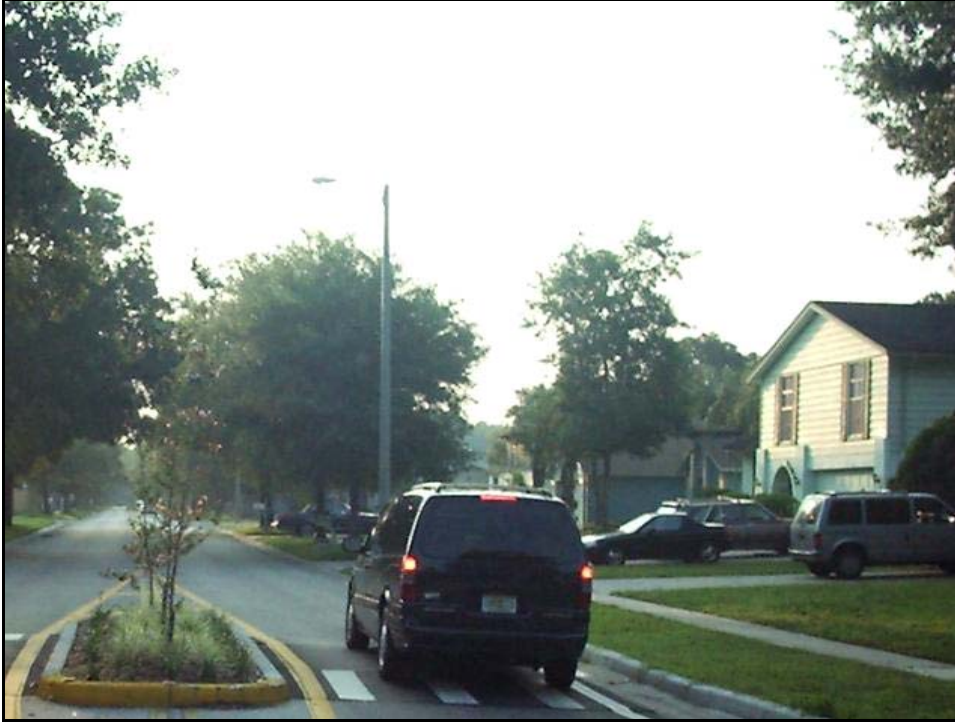
Island in center of residential roadway narrows the cartway
