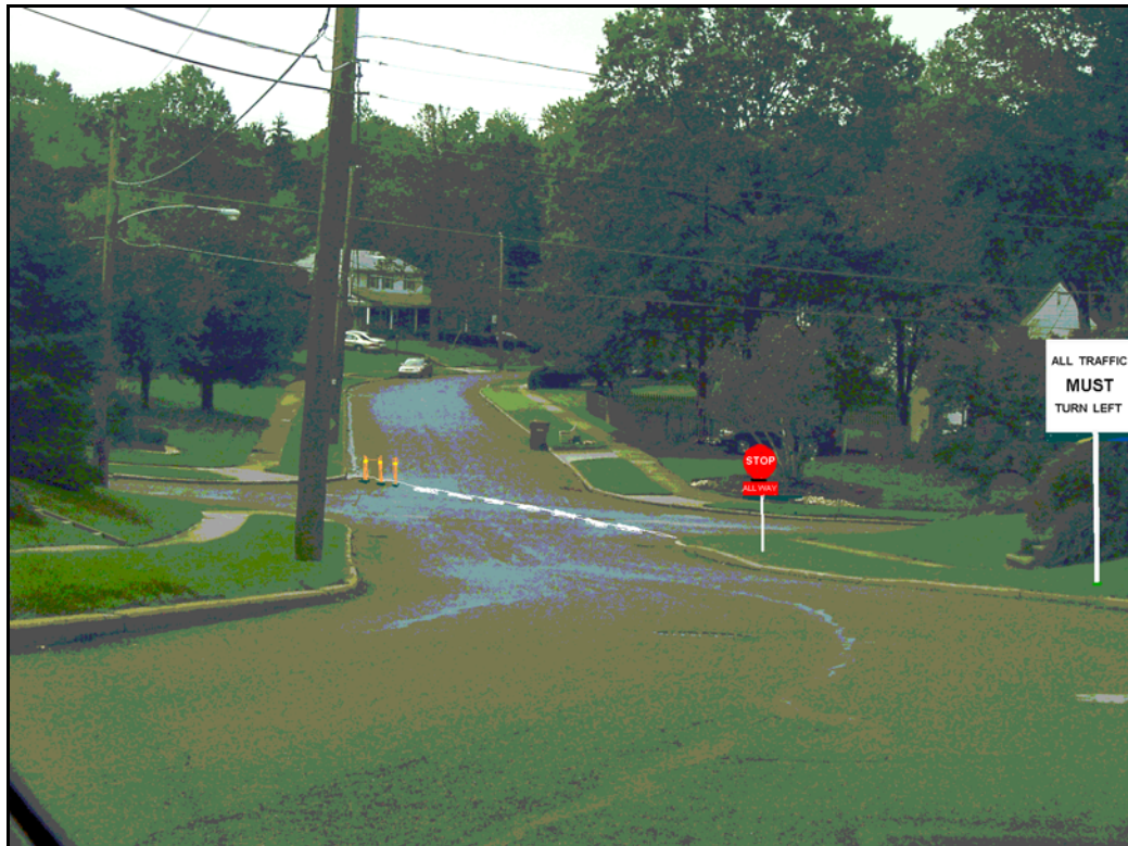
Diverter concept would direct Dundee Drive traffic in both directions to turn left on Burn Brae, with All-Way Stop. Emergency vehicle access through orange flexible posts on left.
