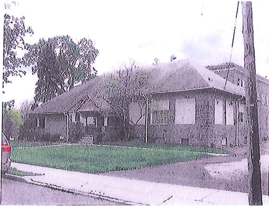
Old Fort Washington School, Building A (circa 1891).
