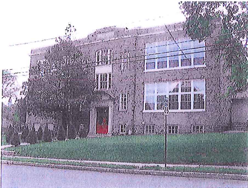
Old Fort Washington School, Building B (circa 1913-1917).
