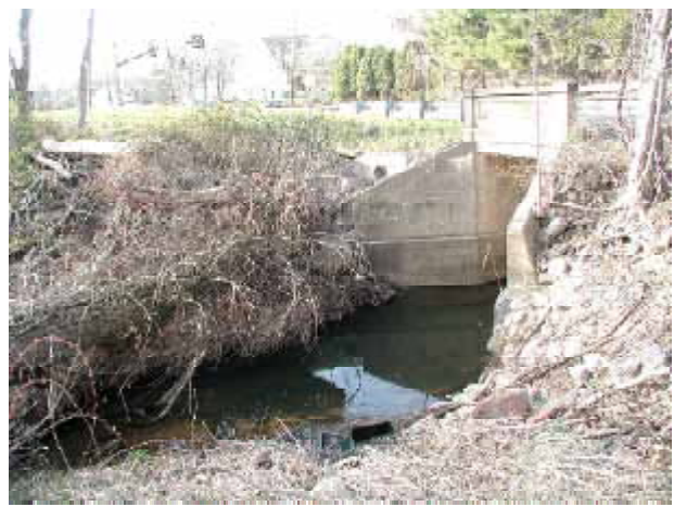
Culvert at creek adjacent to Jarrettown Inn
