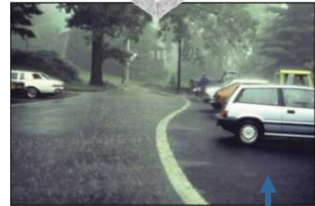
Porous pavement at the Morris Arboretum photo taken during Hurricane Floyd (1999)
