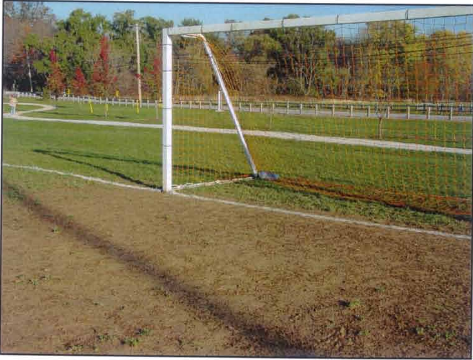
Camphill & Highland (CHAC) South—lighted, high use level, poor condition Fall 2005
