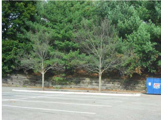
Drainage discharge onto parking lot- New York Drive
