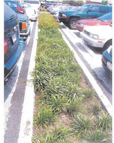
Lined Bioretention Strip in parking area Parking area at Anacostia Navy Yard, Maryland
