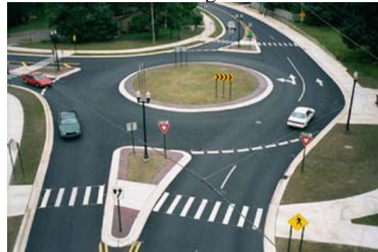
T6B – Traffic Calming with Roundabout
