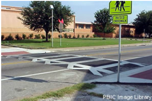
T5A – Raised Crosswalk
