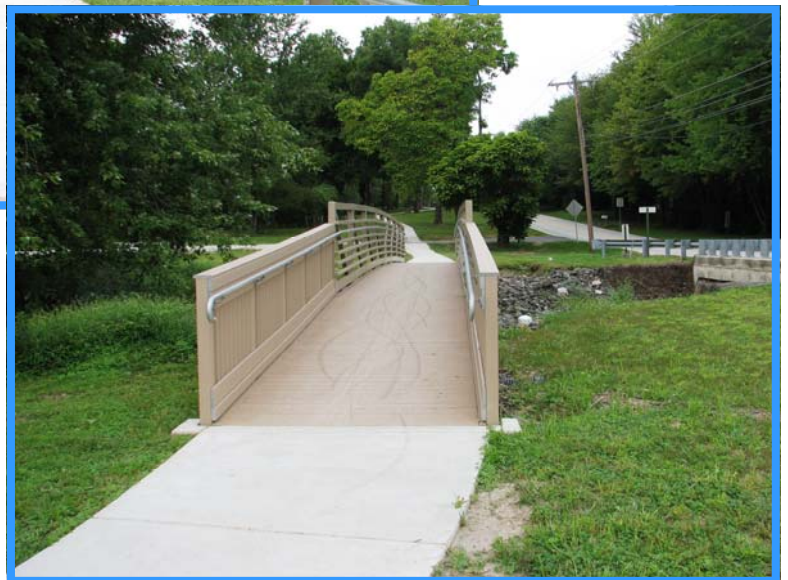
Right - New Trail Bridge over Rapp Run completes sidewalk connection from Ambler Borough to Township's CHAC Complex athletic fields from which pedestrians can then continue on existing CHAC pathways to the future Cross County Trail
