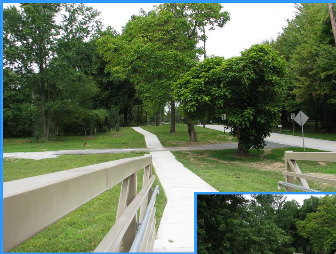
Left - New sidewalk parallels Highland Avenue from existing sidewalk to new trail bridge over Rapp Run
