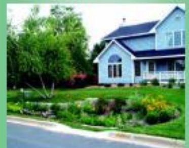
Rain garden with curbside drainage.
