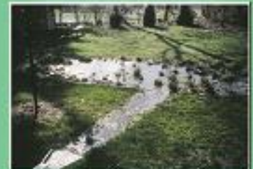
Water heading from downspout to a newly planted rain garden.
