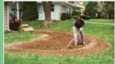
Preparing the planting area next to a roof drain downspout.
